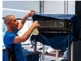
6. In the meantime, use the water lance MGK04AS to clean the framework and the filters left in the floor bag. Use only cold water to clean the filters: hot water causes dust to lump together, lengthening the washing operation.
