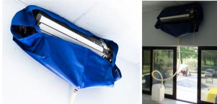
5. Add the "Enzymatic Detergent" into the spray bottle correctly diluted as indicated on the product. Now spray the exchanger battery, and all the plastic and aluminium parts that needs to be cleaned. Leave on the detergent 1 minute.
