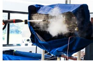
11. Leave the wall bag in place, switch on the air conditioner in fan mode until all the residual water on the fan and the exchanger is dried.
